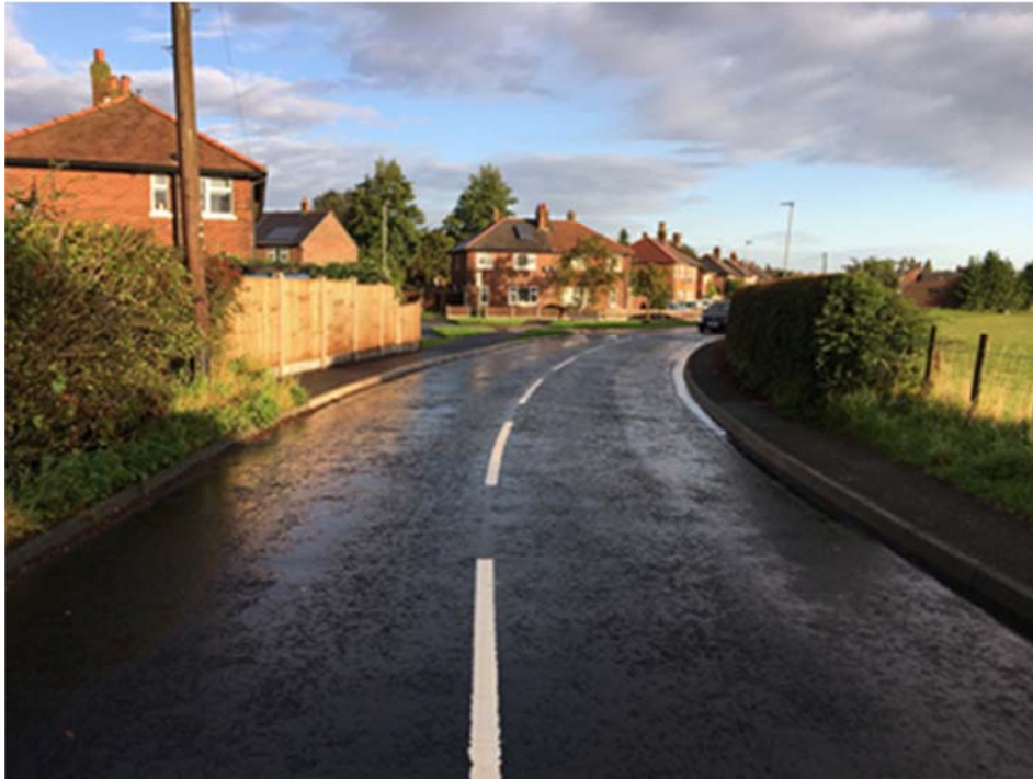
Figure 2 – Raised Table at Haley Road South and Clay Lane Junction
