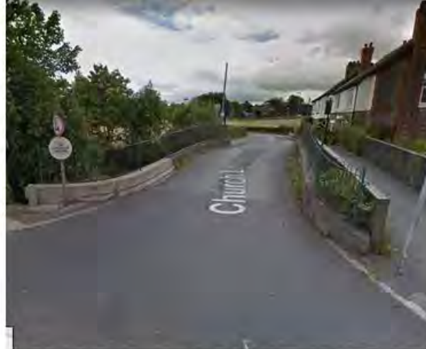
Stanney Lunt Bridge and Church Lane from A56 Chester Road looking towards proposed development
