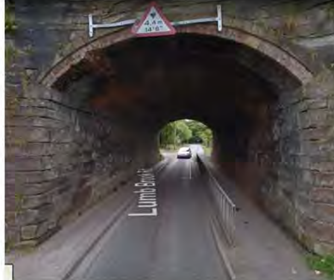
Lumb Brook Rd underbridge (view approx. south toward proposed development)
