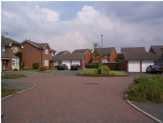
Figure 27: Typical Cul-de-sac Turning Head
