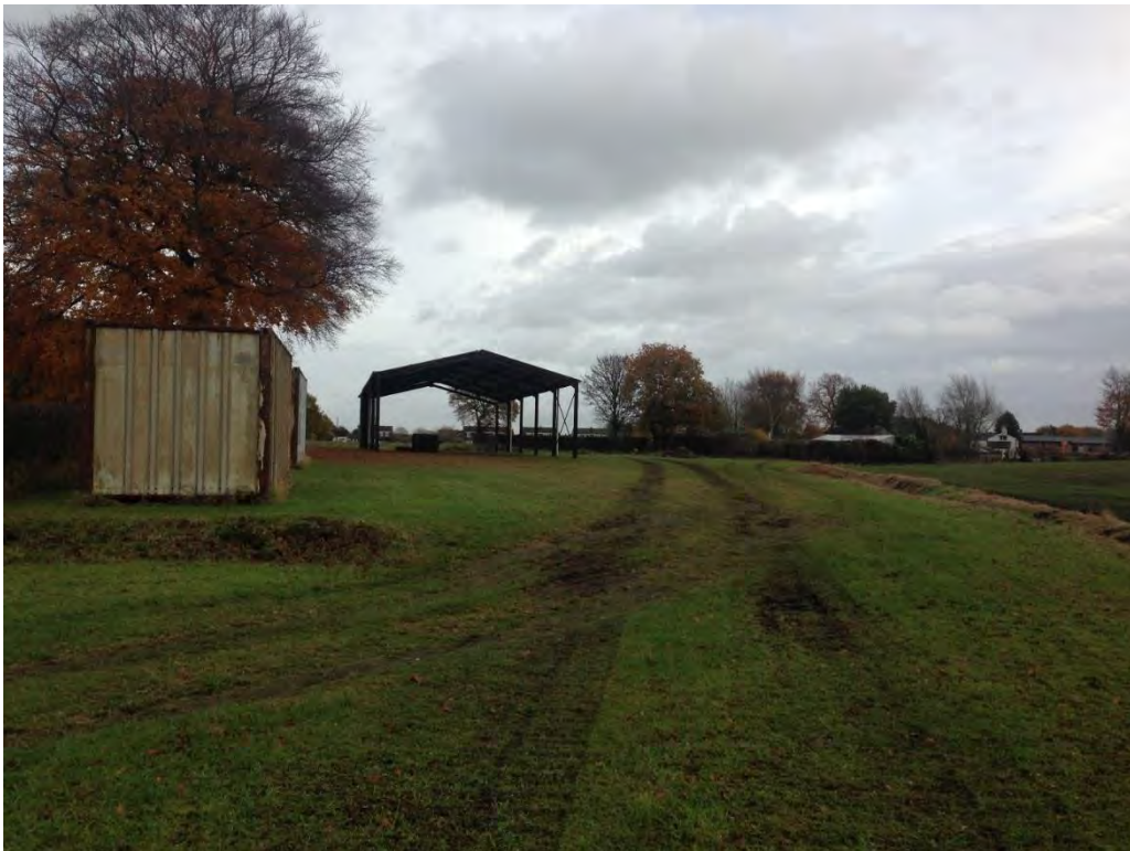
7. View looking eastwards towards existing agricultural buildings.
