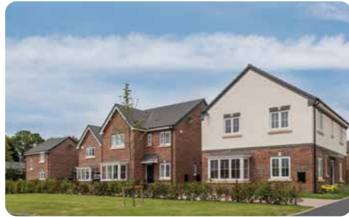
Development will promote a low carbon lifestyle through the consideration of the environmental performance of buildings. (Miller Image)
