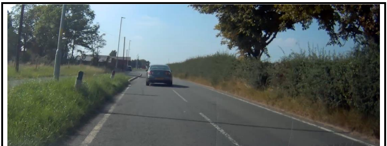
Northbound away from Tan House Lane junction and shared path running alongside carriageway.
