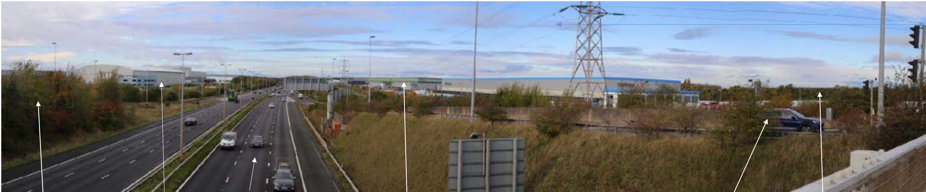
M62 structure planting Omega South warehouses M62 Eastbound Brakes and Hermes logistic centres Eastbound Jnc 8 slip road leading to overbridge Structural tree planting
