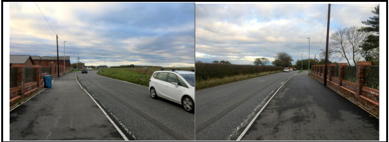
View away and to access location on NW side
