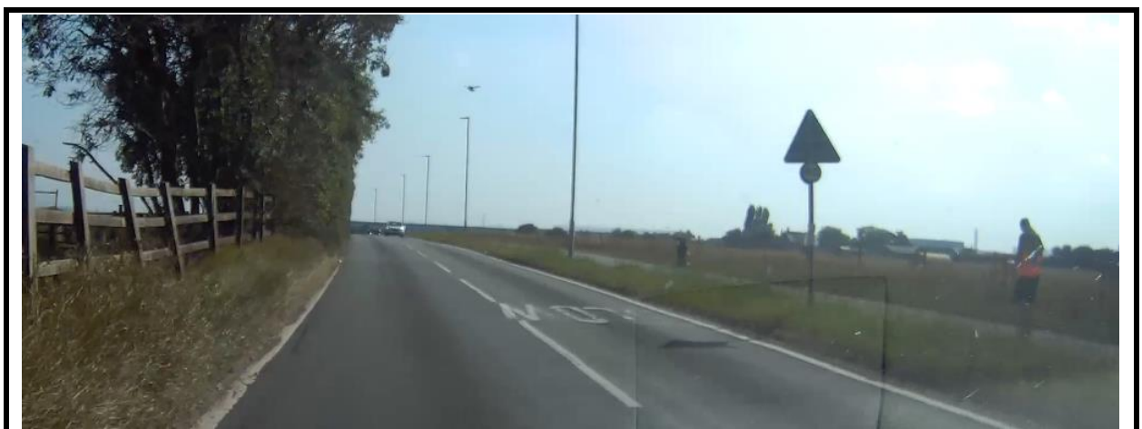
Heading south from village/bend towards site
