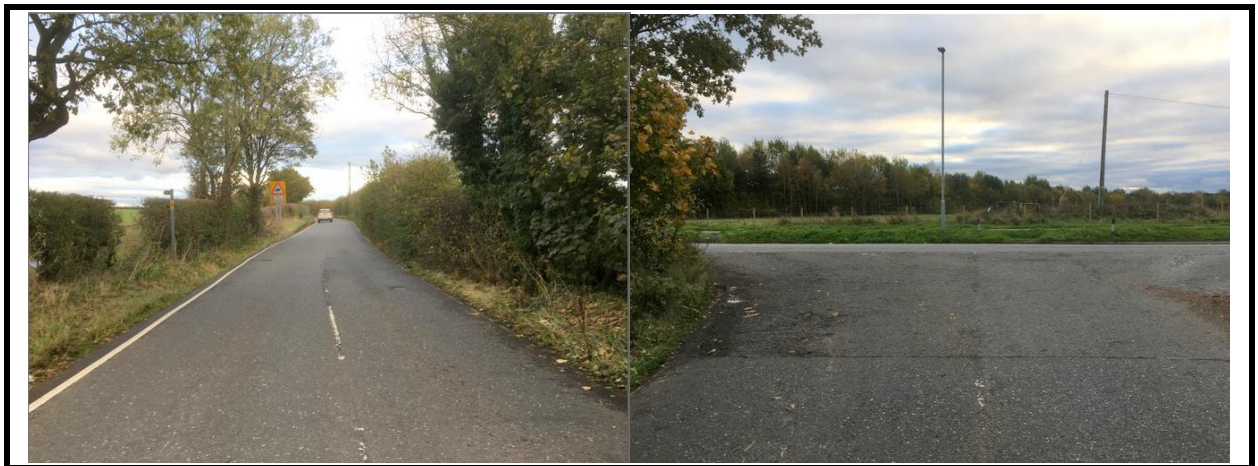
Tan House Lane away and to Junction with Burtonwood Road
