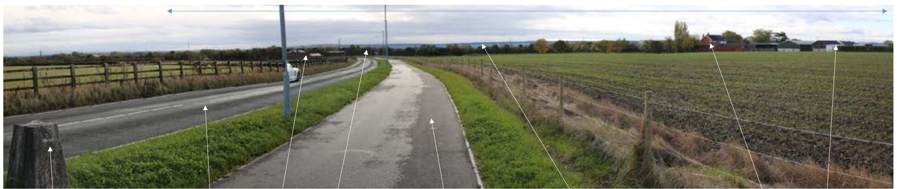
Trig Point marking high point of shallow local ridge Clay Lane Finger Post Farm Structural tree belt New Burtonwood to Omega North cycle link Hermes warehouse Open field sides Highfield House and farm buildings
