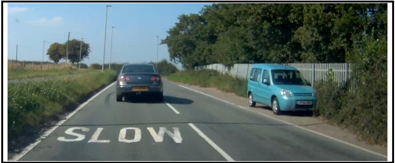
Traveling north showing shared cycle walk path and street lighting, slow markings to left hand bend.
