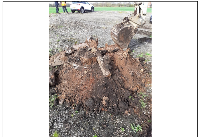
Trial Pit 119 Spoil
