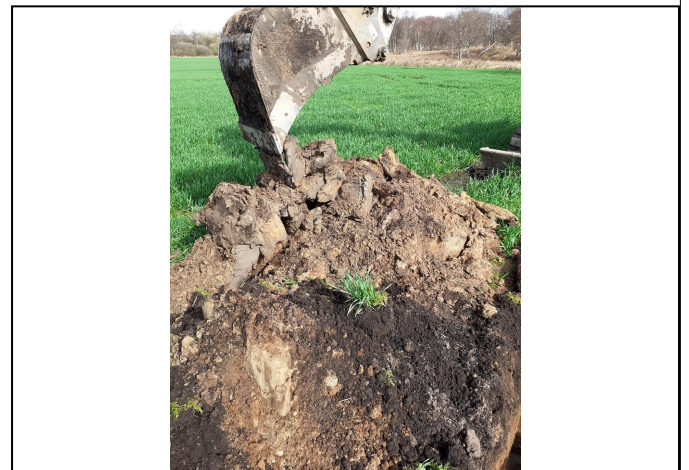
Trial Pit 123 Spoil
