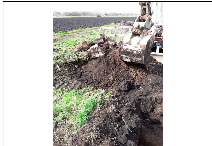
Trial Pit 109 Spoil
