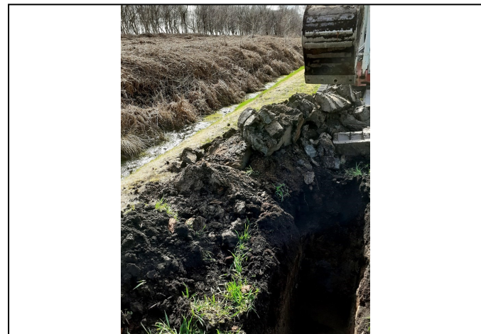
Trial Pit 122 Spoil
