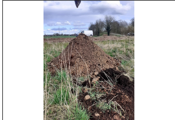
Trial Pit 130 Spoil
