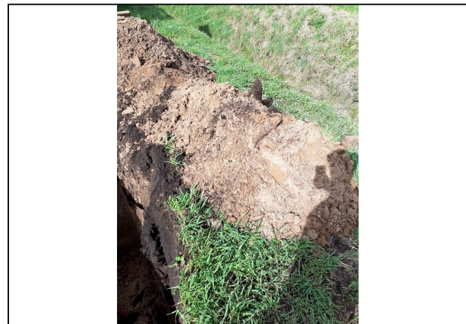
Trial Pit 125 Spoil
