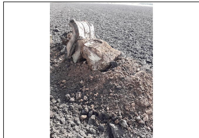
Trial Pit 110 Spoil
