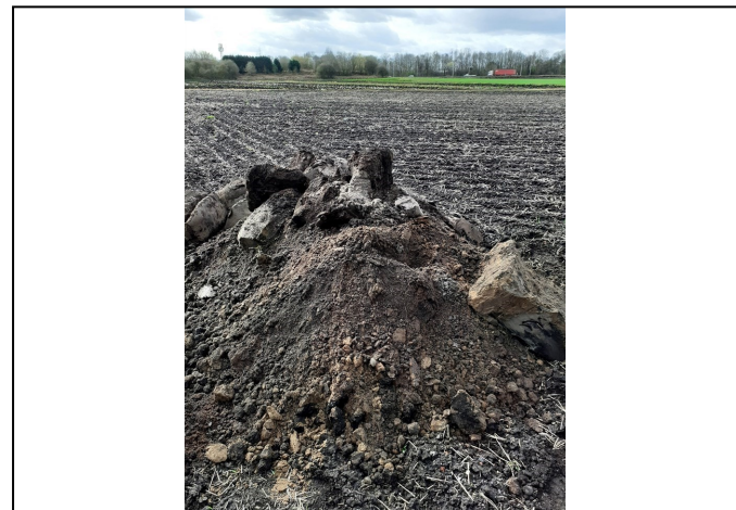
Trial Pit 107 Spoil
