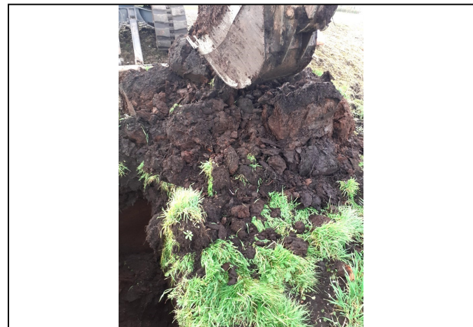
Trial Pit 129 Spoil
