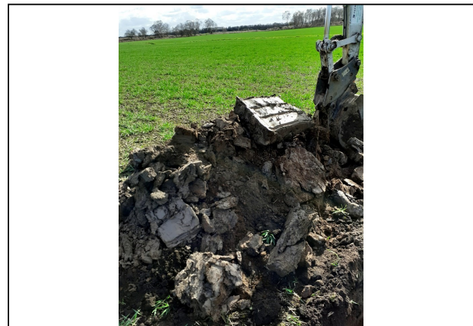
Trial Pit 121 Spoil
