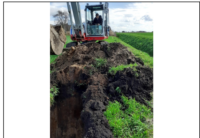
Trial Pit 124 Spoil
