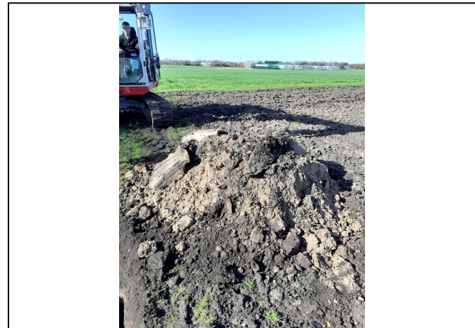
Trial Pit 115 Spoil
