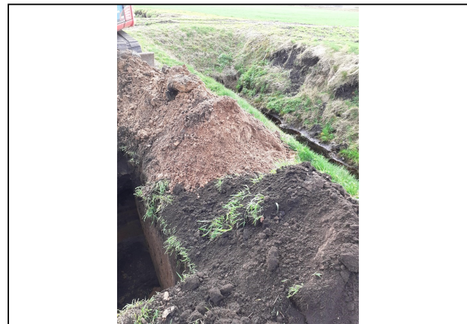
Trial Pit 120 Spoil
