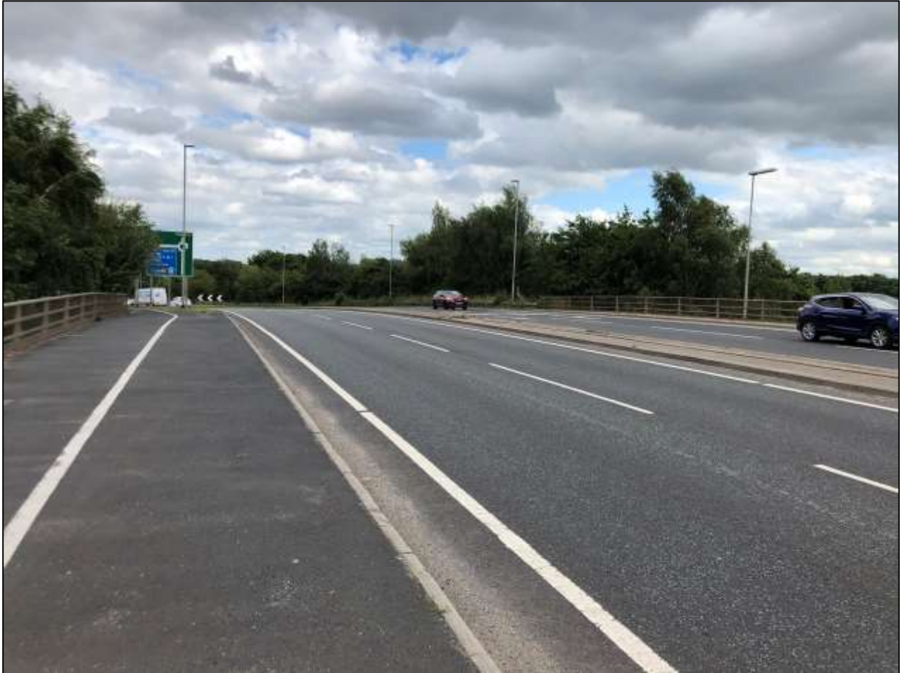
Figure 3.3: Shared Footway / Cycleway Route on A57 Manchester Road at the M6 Junction 21
