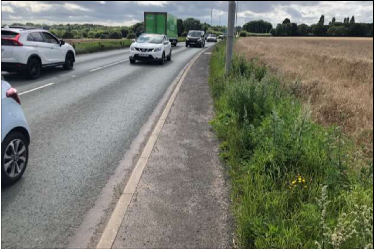
Figure 2.5: A57 Manchester Road Adjacent to the Site Looking West
