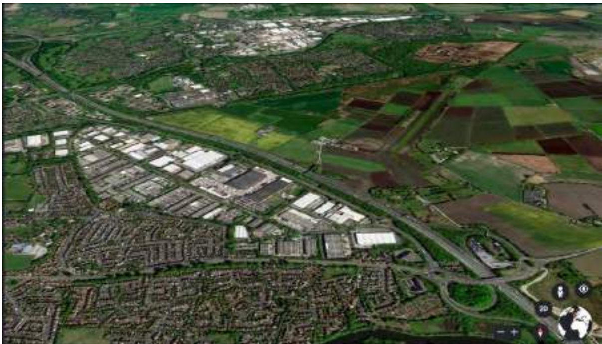
Figure 6: Aerial Image Illustrating the Urban Landscape Context to the North and West of the Site
