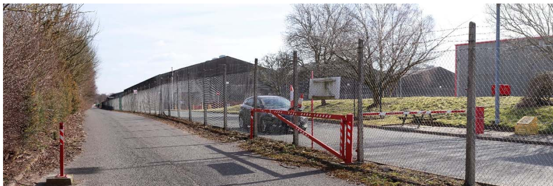
Landscape Photograph 1 - Existing buildings at Port Warrington
