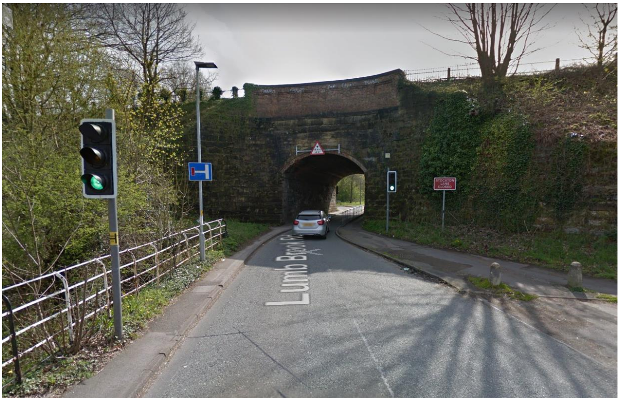
Lumb Brook Rd underbridge (view approx. south toward proposed development)
