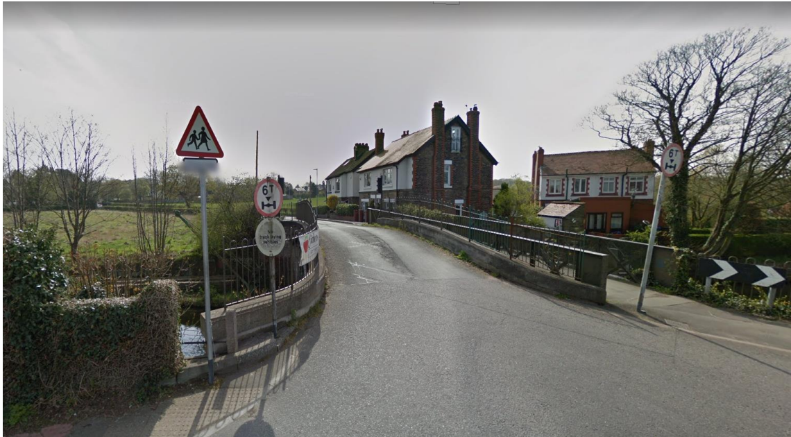
Stanney Lunt Bridge and Church Lane from A56 Chester Road looking towards proposed development (Note, single track, traffic lights controlling junction and 6t axleload restriction)
