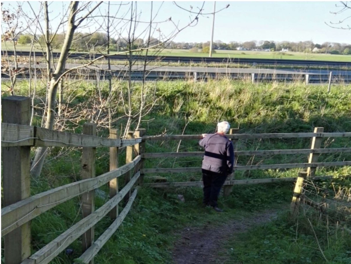
Public Right of Way – 2.5 metres below M62 motorway
