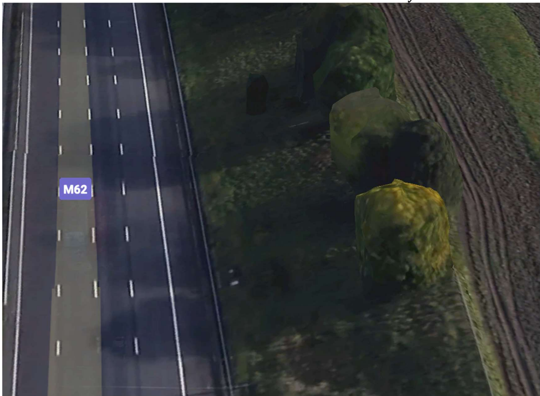
Embankment - 25 meters width - 7.5 meters above motorway
