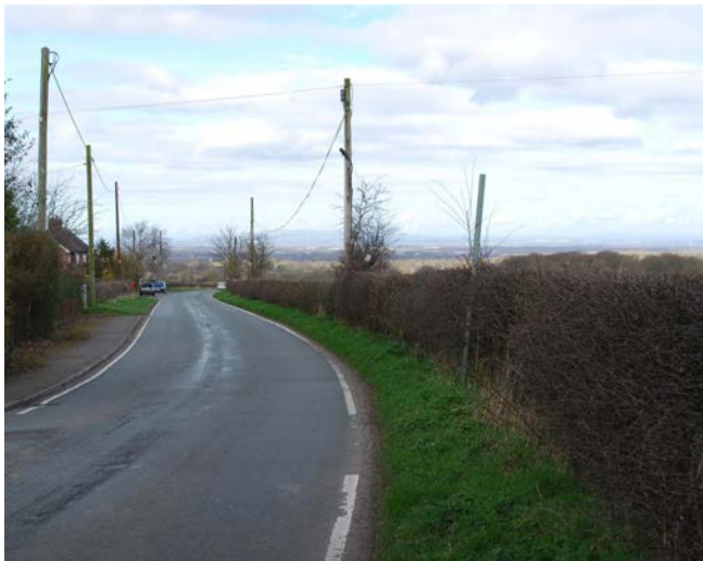
Existing view of Broad Lane
