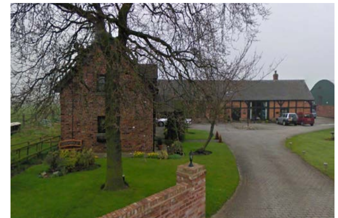
Grade II* Listed Tanyard Farm building
