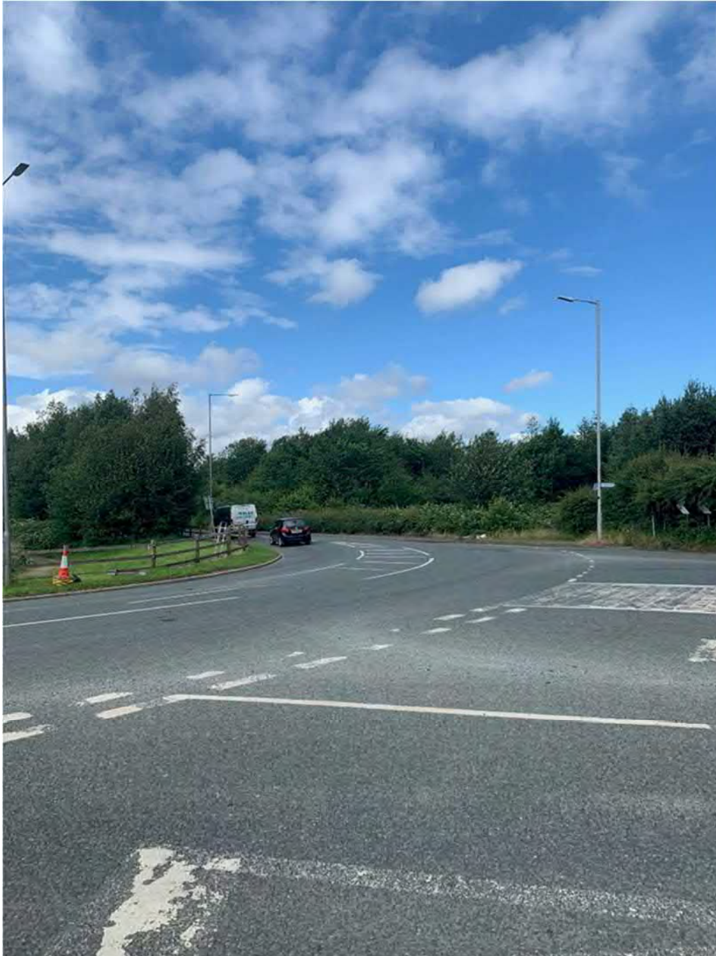
Figure 3-10 - Poor visibility on the bend due to overgrown vegetation
