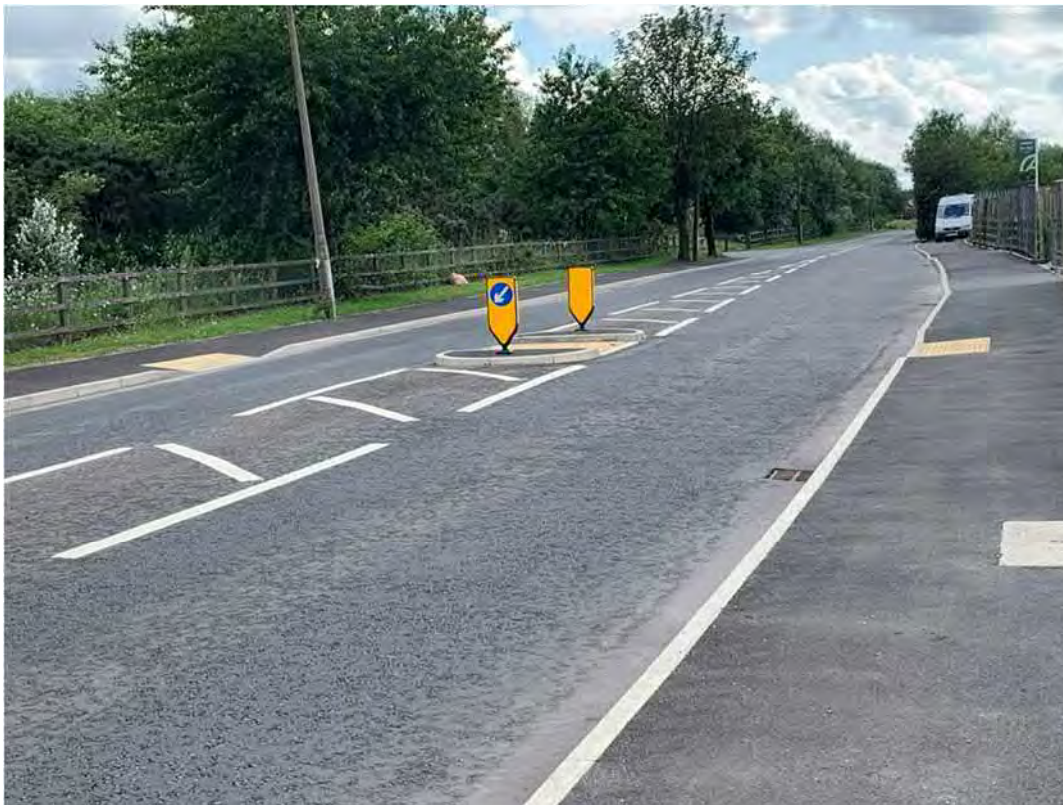
Figure 3-22 - New crossing with tactile paving
