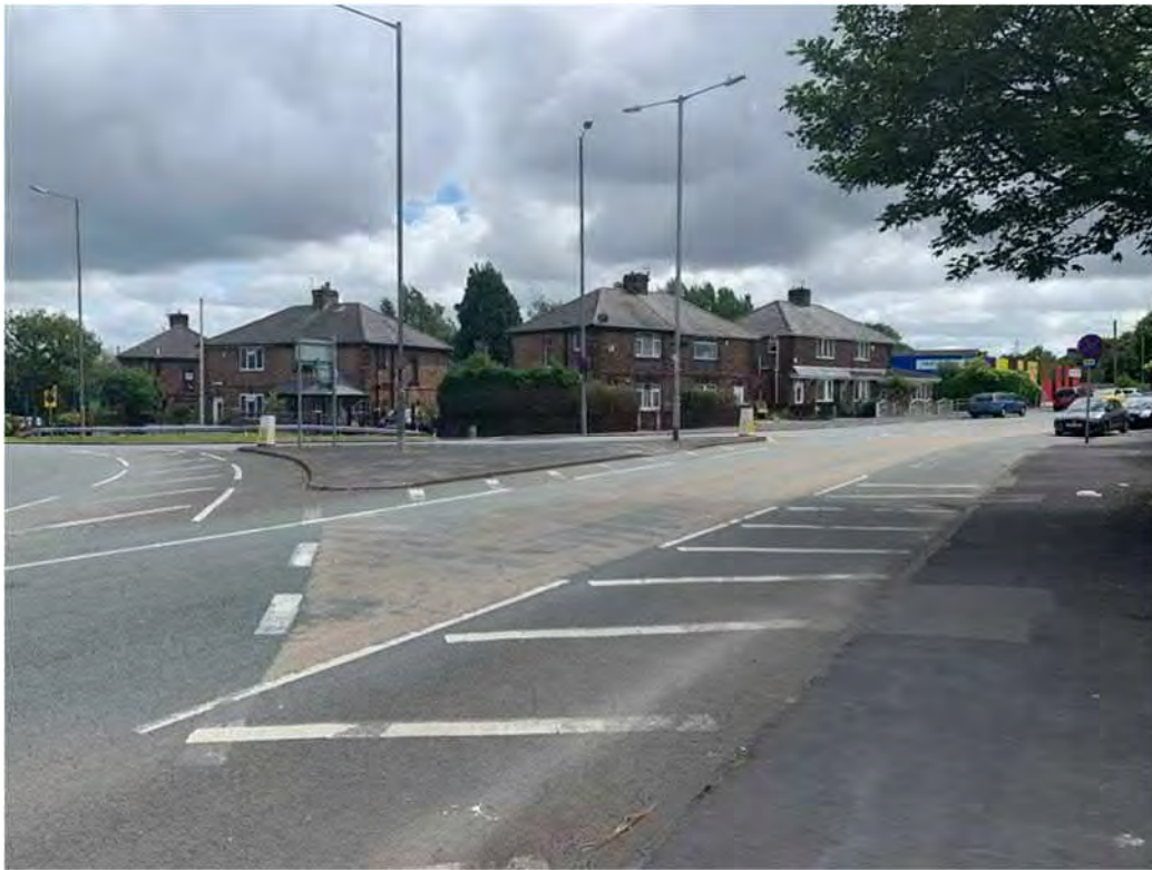
Figure 3-4 - Pedestrian crossing at the roundabout - dropped kerbs but no tactile paving
