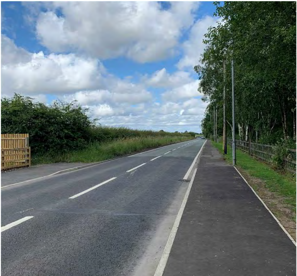
Figure 3-20 - Footway on south side
