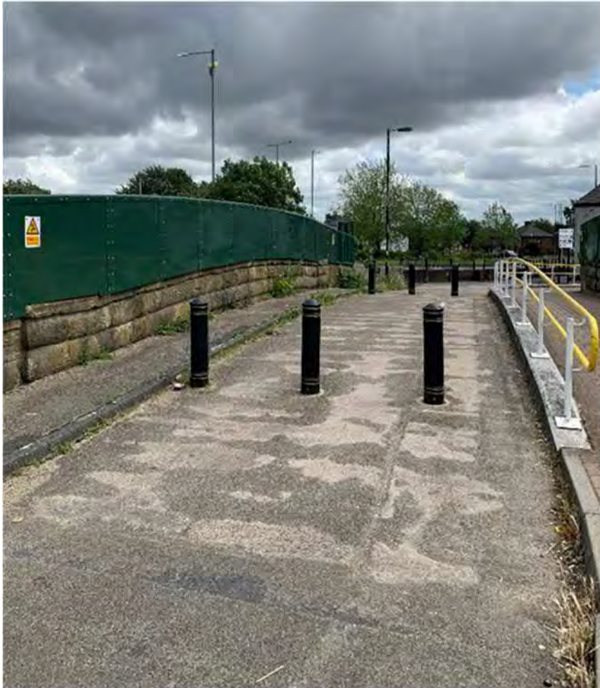
Figure 3-30 - Bollards preventing vehicles accessing this road
