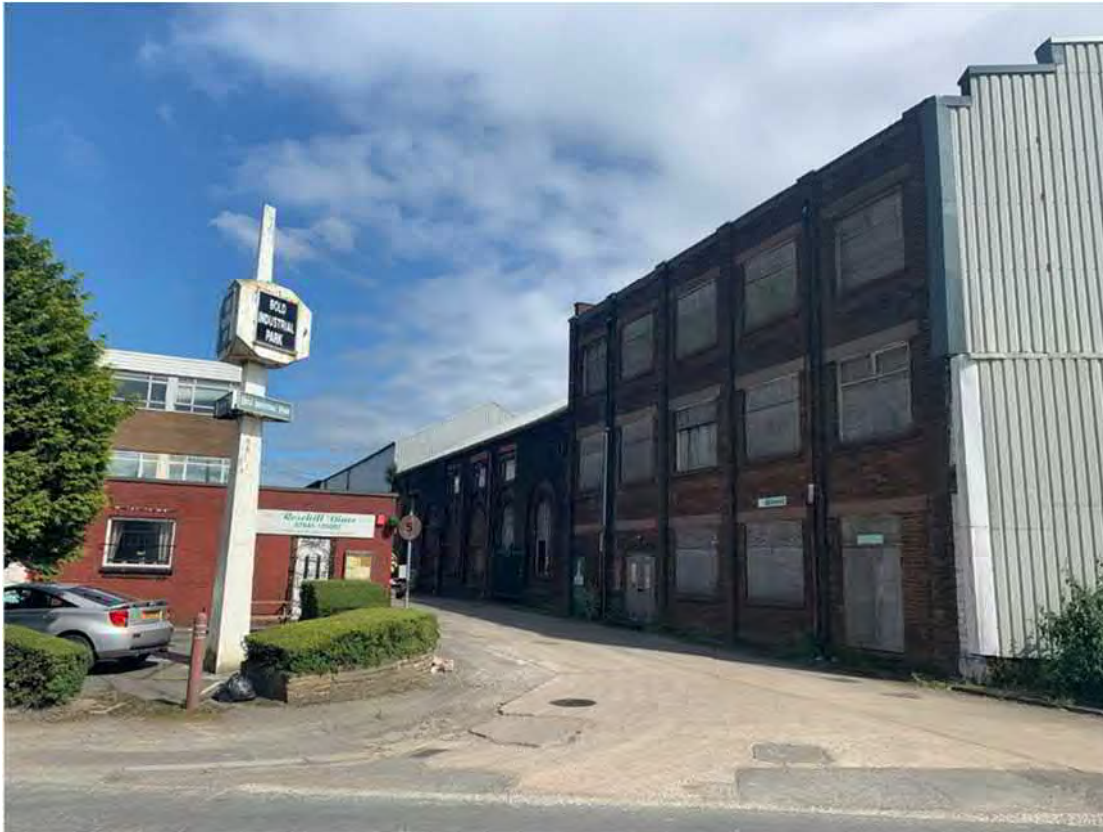
Figure 3-13 - Industrial Site and Car Park Entrance
