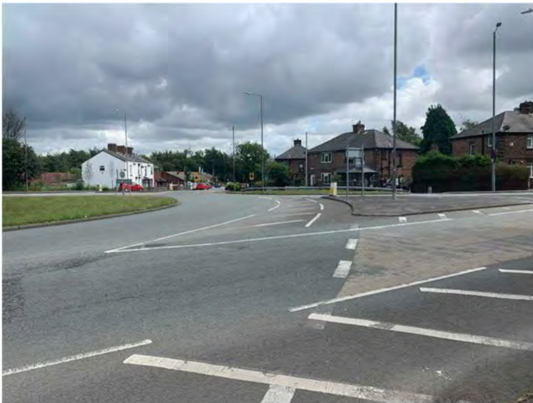
Figure 3-2 - Wide lanes at the roundabout near the Bull & Dog Pub
