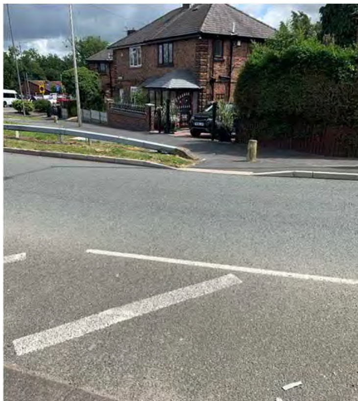
Figure 3-4 - Pedestrian crossing at the roundabout - dropped kerbs but no tactile paving
