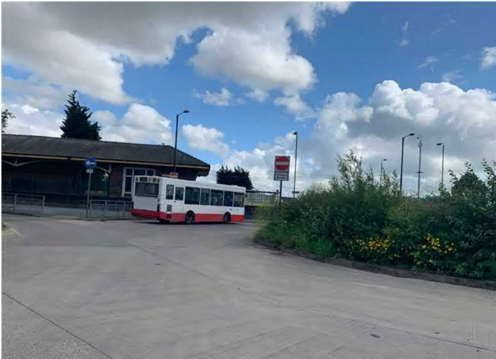
Figure 3-35 - No entry sign except for buses and overgrown vegetation
