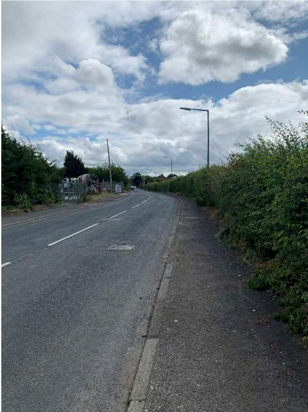
Figure 3-12 - Poor visibility due to overgrown vegetation and bends
