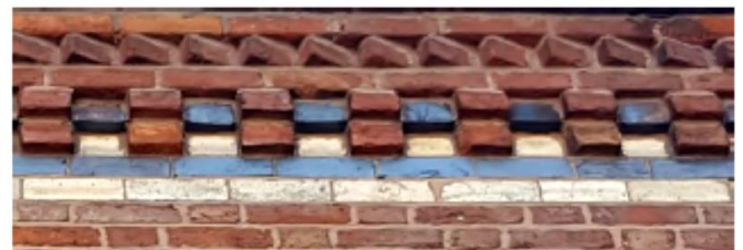
Brick cornice detailing 21 Bold Street
