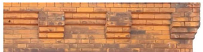
Brick cornice detailing 12 Bold Street
