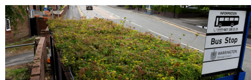
Bus Shelter Improvement Programme 2023-24
