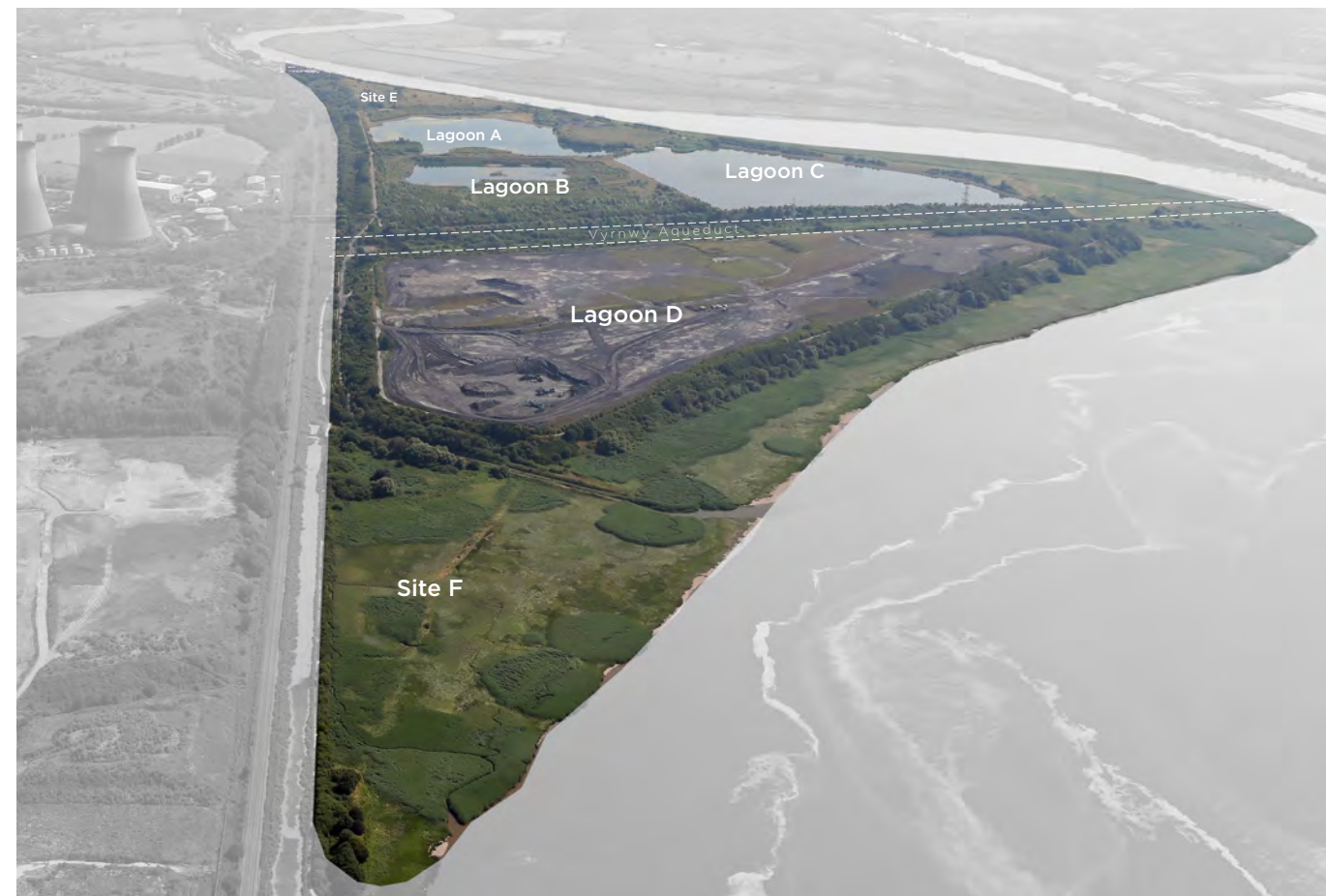
Land south of the rail line Summer 2021
