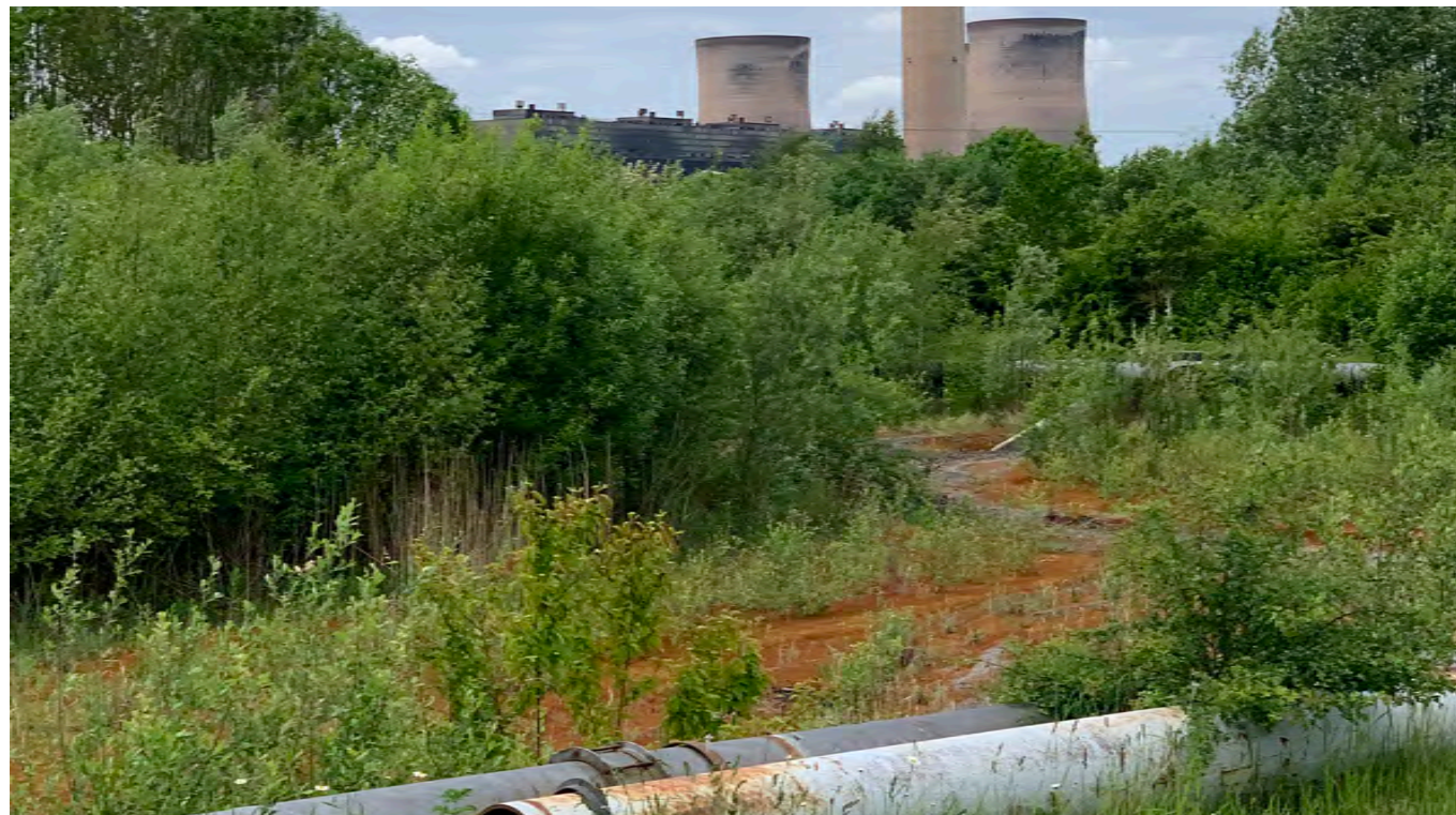
Existing lagoon area south of the rail / canal corridor
