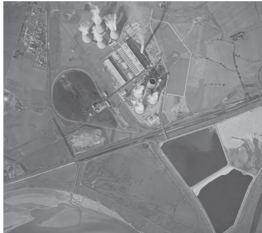
Historic photograph of Fiddlers Ferry Power Station operating shortly after construction showing original landscape context (image date unknown)
