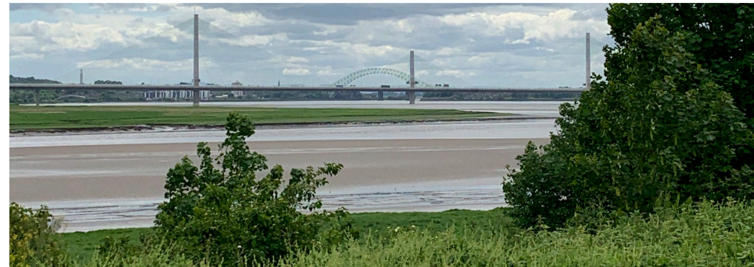
View out from the lagoon area towards the river foreshore and bridges
